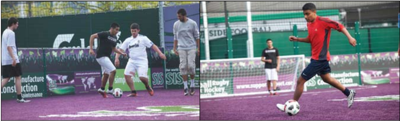
SIS rose to the challenge with the construction of a two-tiered pitch layout, which also saw the installation of a UK-first in the form of a demountable fencing system, which has been specifically designed for the site, utilising removable modules to provide a more open plan profile to pitches during events.
